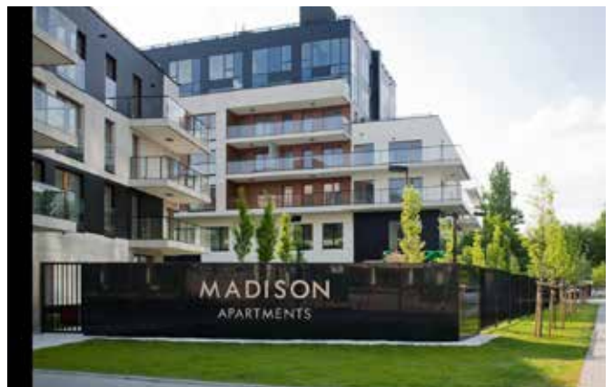
Madison Apartments - Polonia - Clima Canal
