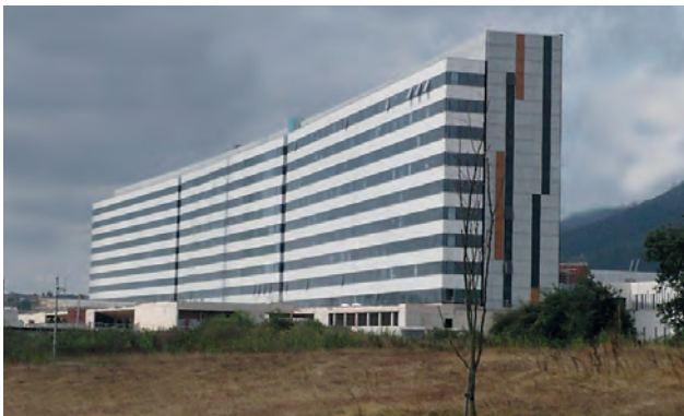
Hospital Central, Asturias
